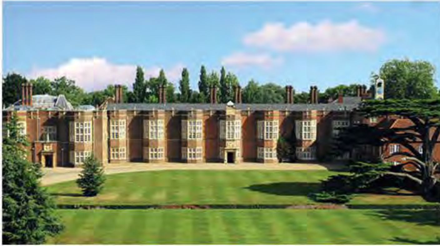
New Hall School, Chelmsford
