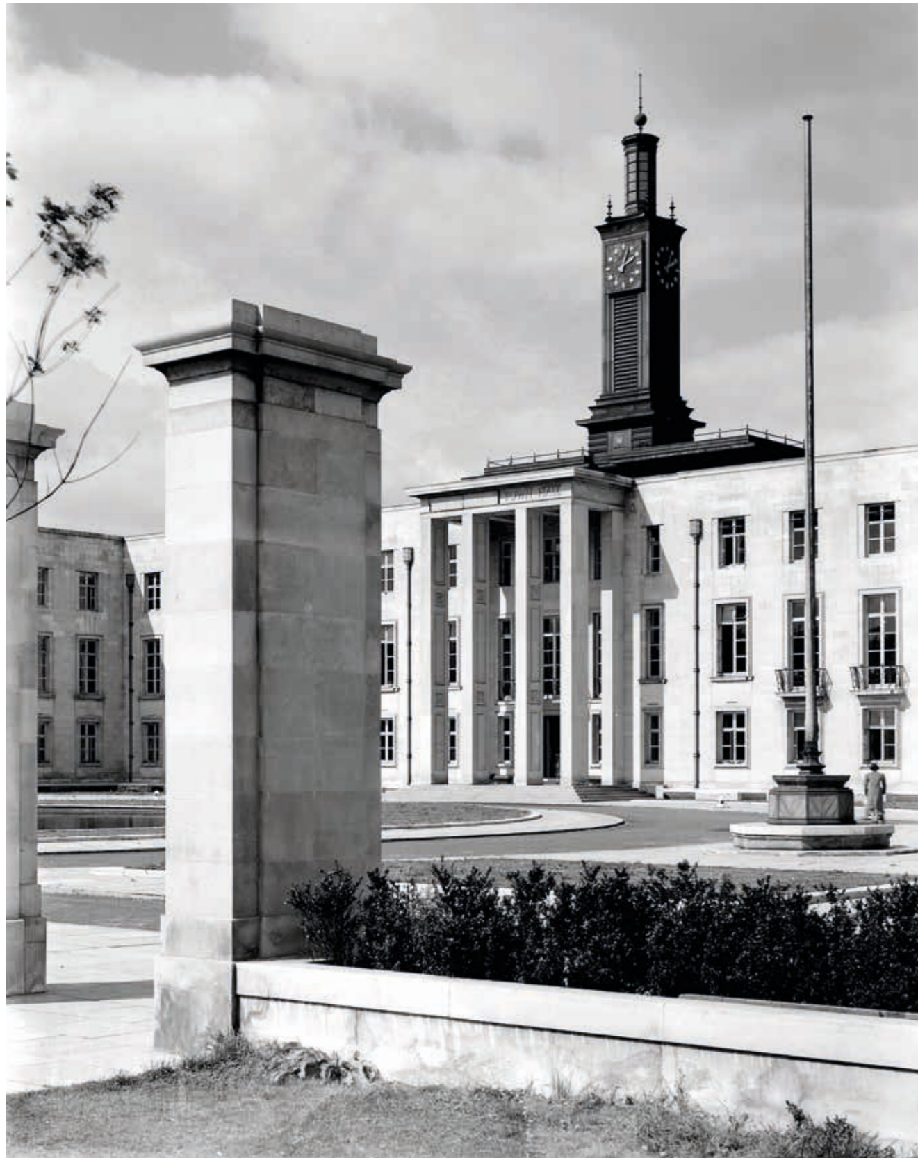
Town Hall, Walthamstow
