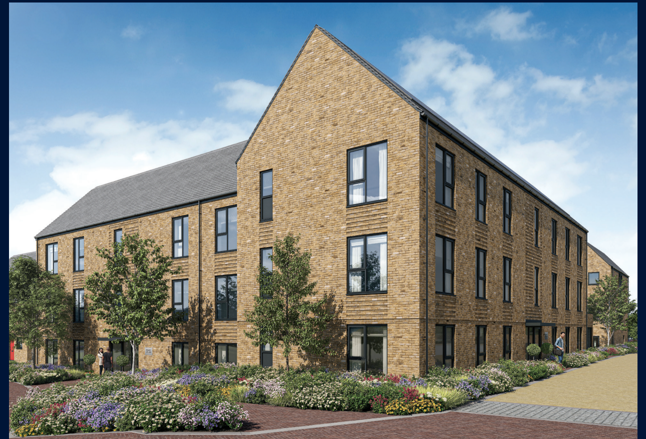
Computer generated image of The Nova Apartments
